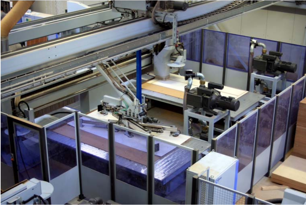
Fig. 3: Cell 1 HOMAG processing centre with direct loading from the panel store
