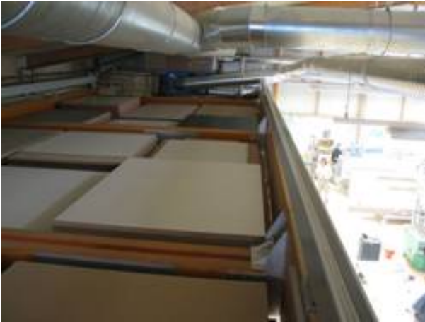
View from the storage area to the production hall
