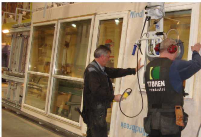
Montajul ergonomic al ferestrelor / Ergonomic installation of window elements
